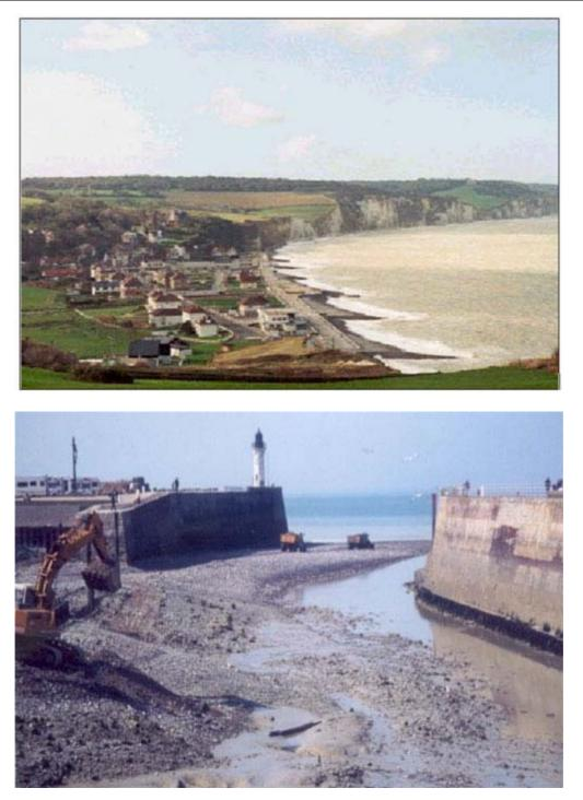
Fig. 12a & 12b: Hard protection on photo A (Pourville) and soft (B) (extraction of the pebble on the harbour and put it on the beaches (Saint-Valéry en Caux).
