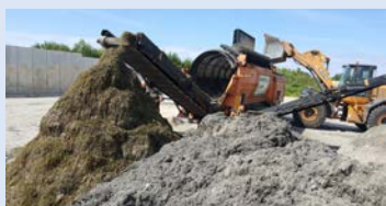
Case Study 1 Soil improvement products, Bad Doberan/Poel, Germany
