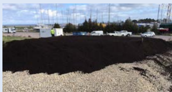
Case Study 3 Compost for methane-mitigating biocovers, Køge Bay, Denmark
